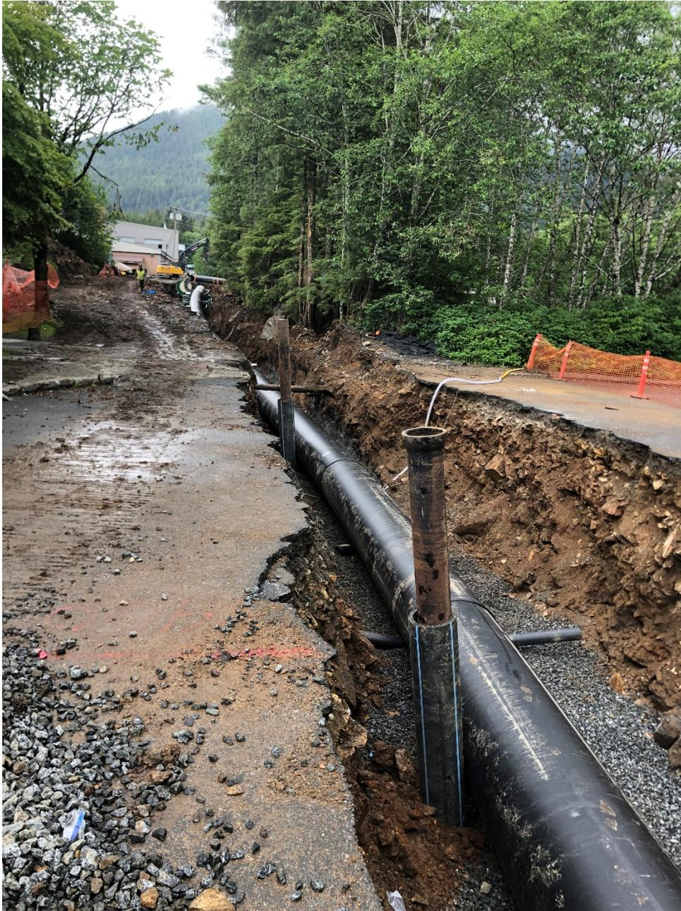
Once it is installed in the new trench and connected to the existing 240-foot segment of HDPE pipe with an electrofusion coupling, the entire exposed length will be backfilled. It is first completely bedded with fine gravel all-around to provide uniform support and then backfilled with larger material to finish grade, and finally compacted.
